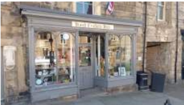
Timber shopfront with stone base to stallriser
