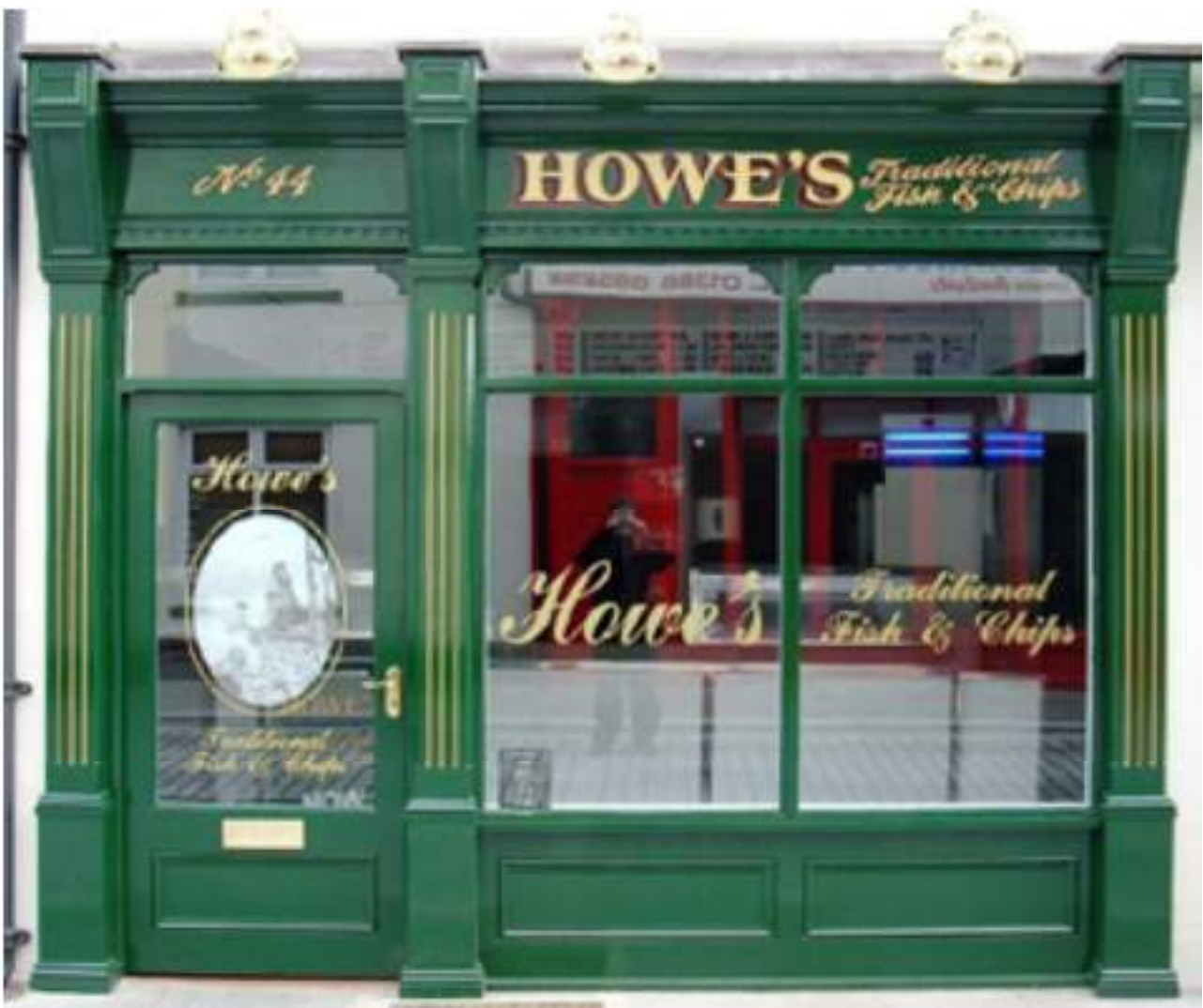
Shopfront featuring traditional materials, architectural detailing and hand-painted signage
