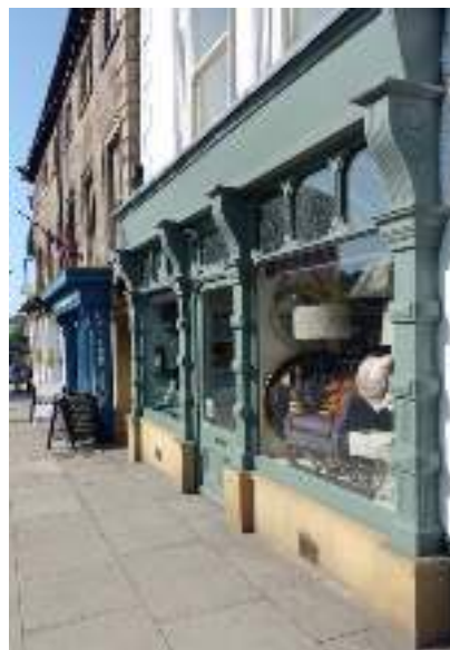
Level access into a highly detailed timber shopfront
