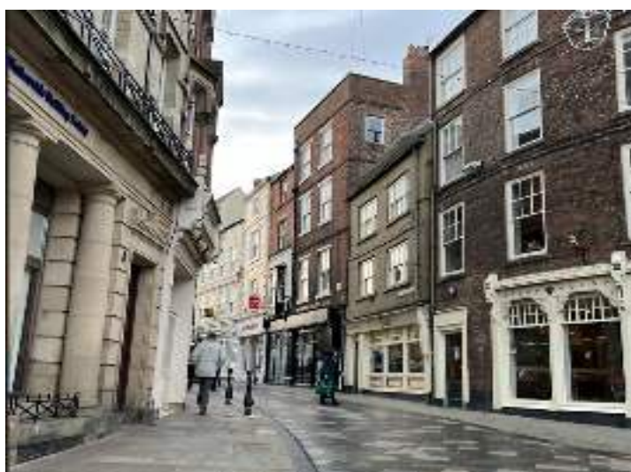
Historic shopfronts lining Silver Street in Durham City Conservation Area
