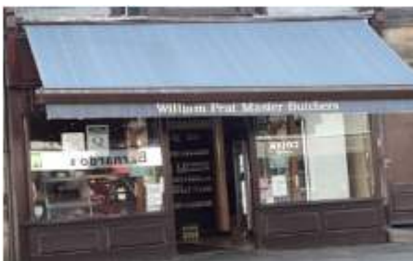
Retractable canopy above a shopfront
